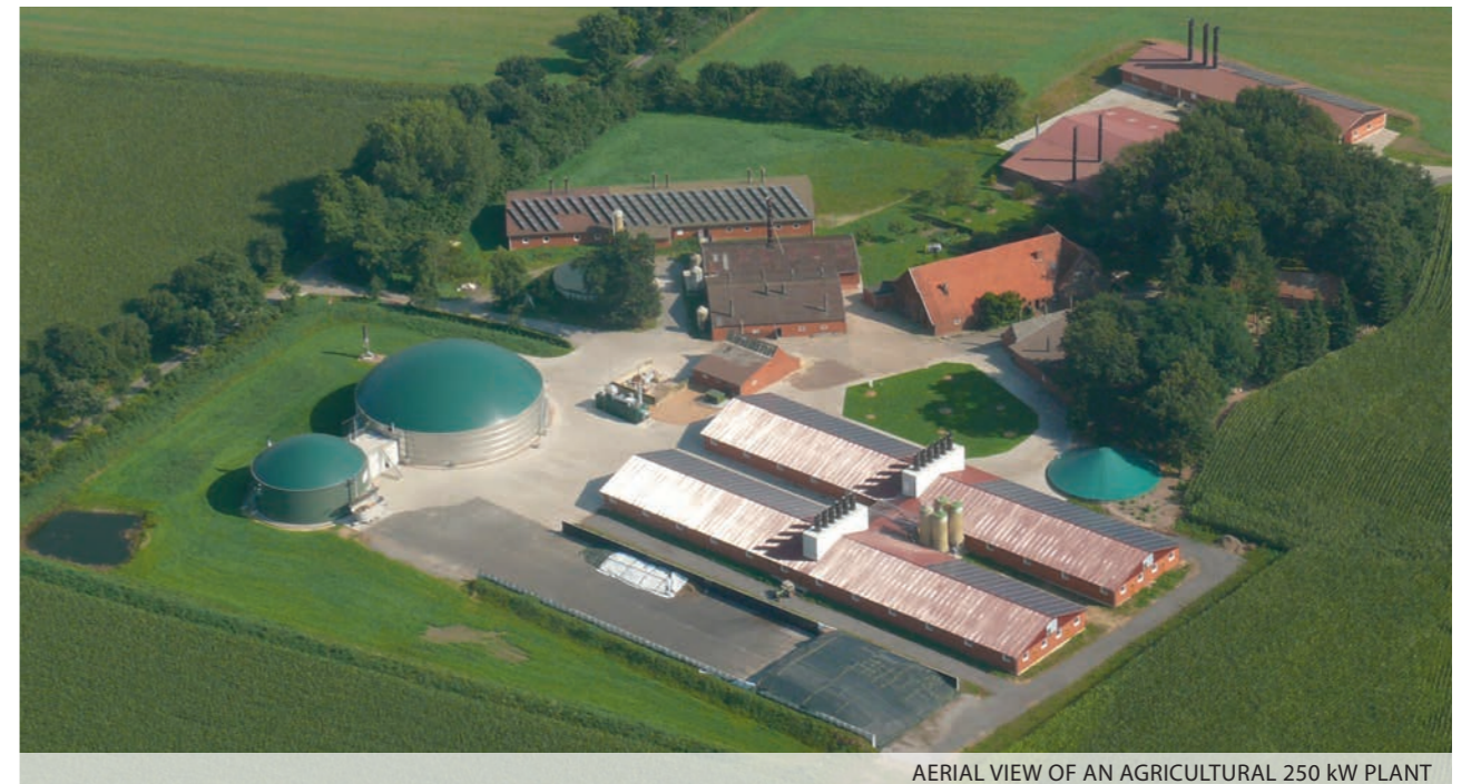
AERIAL VIEW OF AN AGRICULTURAL 250 kW PLANT
