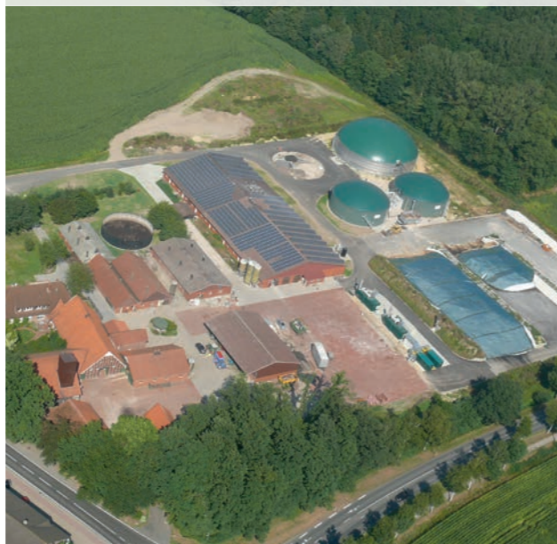
Vechta, Germany Output 770 kW
